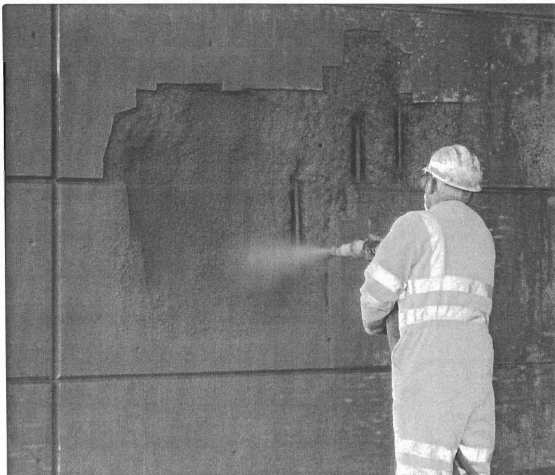
Figure 5: Application of sprayed concrete.
